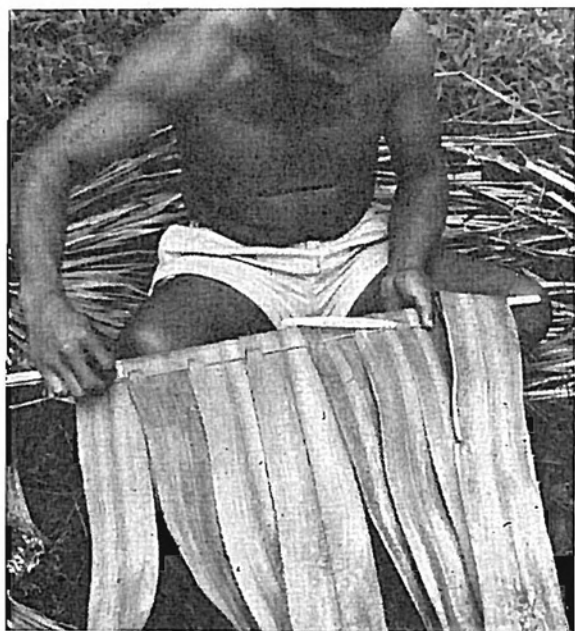
Fig. 47. A thatch panel, mataangan , is made by folding pandanus leaves over a stick. The leaves are firmly secured by being pierced with a midrib from a coconut palm leaf.
